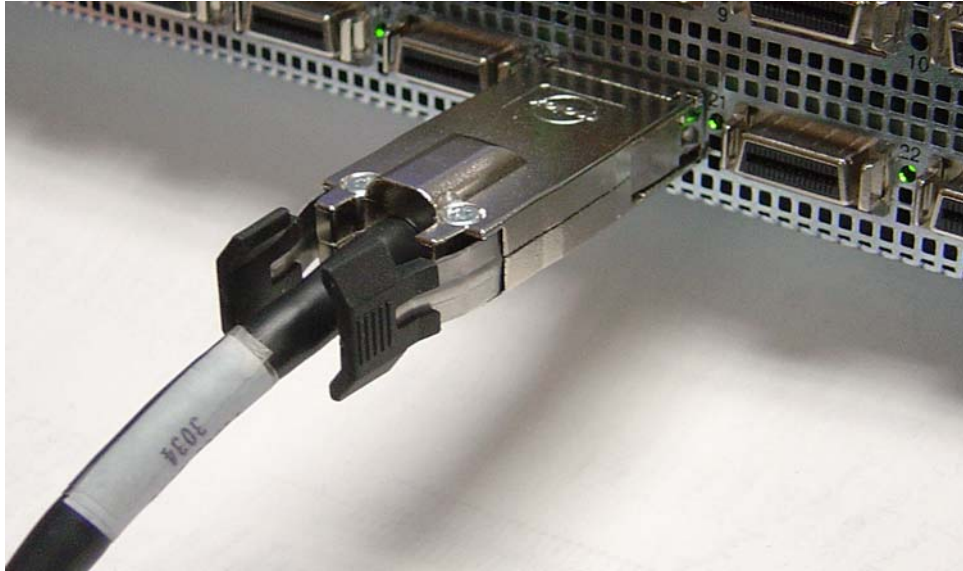
Figure 3-9: Fully Installed IB Cable with Pinch Connector
